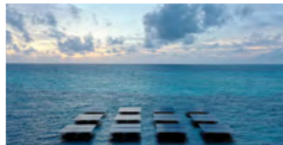
The current floating solar installation at the resort will soon be expanded with additional platforms.
